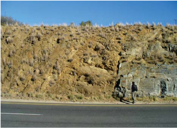
A geological discontinuity, with layered shale on the left and a dolerite intrusion on the right. Groundwater occurrence and movement is enhanced by structures such as these.
