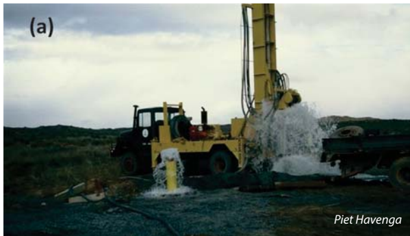
A cement block around a completed borehole prevents contamination from the surface.
