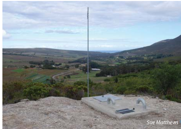
A cement block around a completed borehole prevents contamination from the surface.
