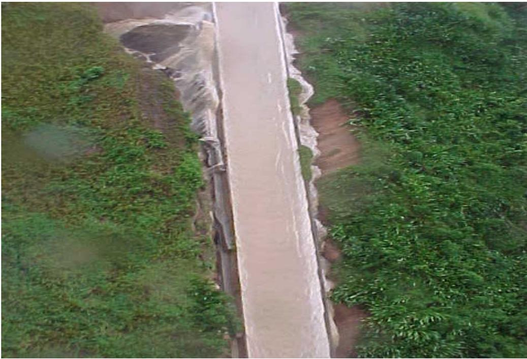
Figure 15: Overtopping of Upstream Chute Walls
