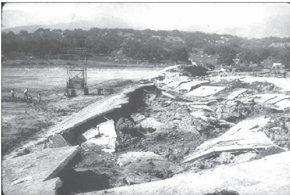
Figure 11: Sheffield Dam after seismic failure
