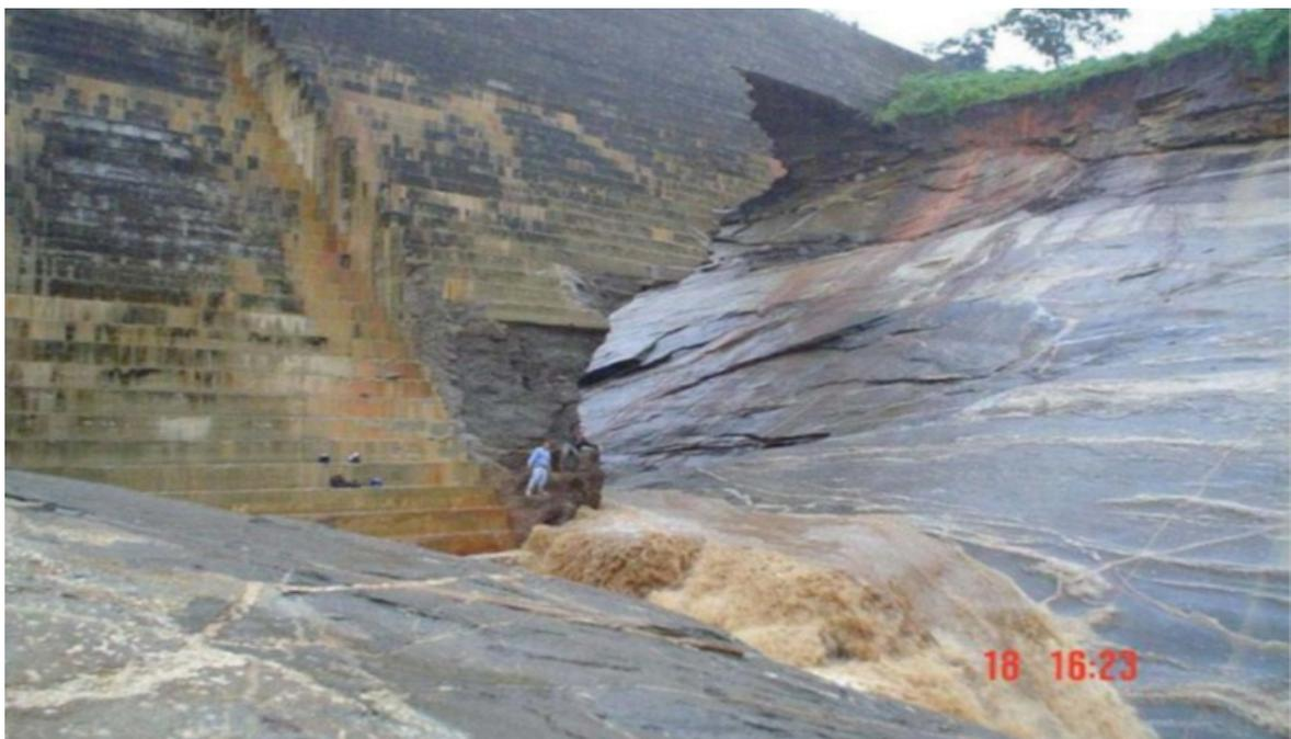
Figure 26: Camara Dam after failure
