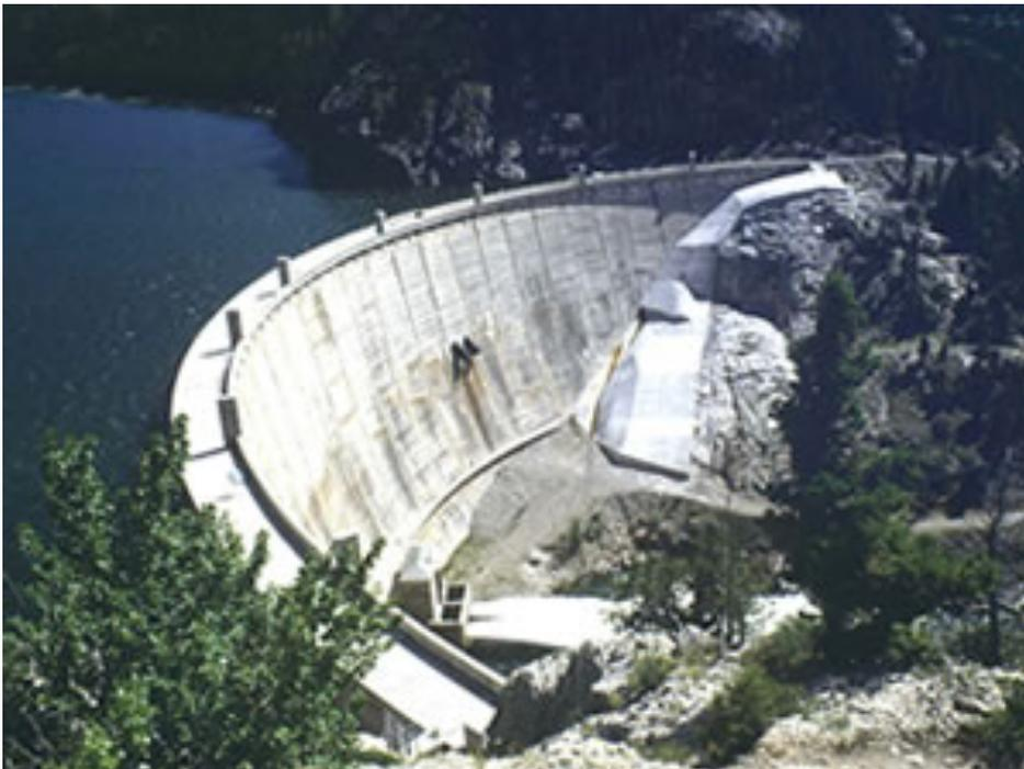
Figure 21: Gibson Dam after some remedial work
