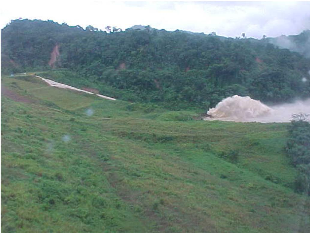
Figure 13: Sweepout of spillway stilling basin
