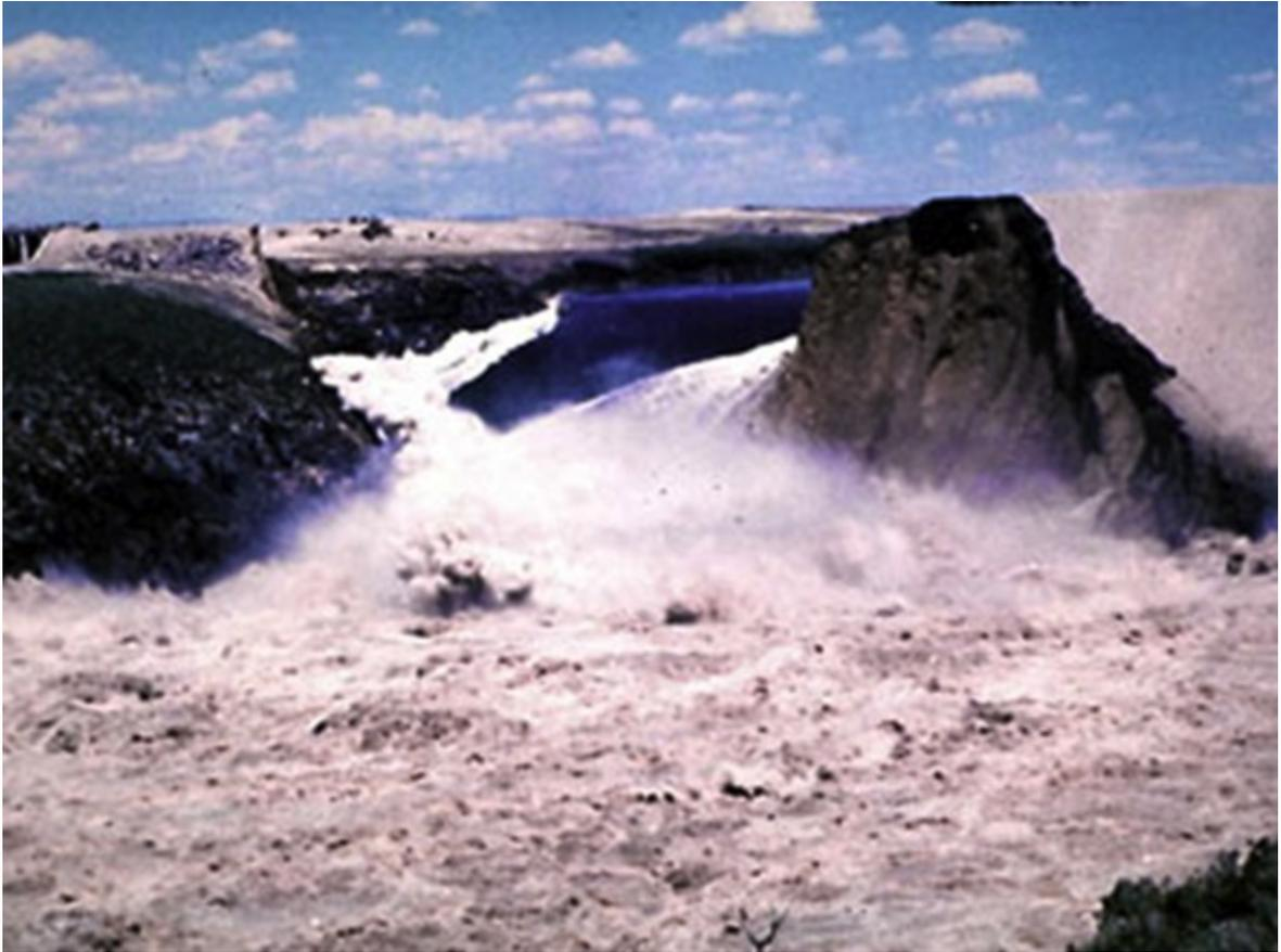
Figure 6: Teton Dam during failure
