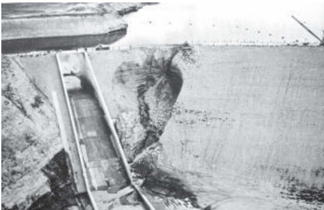
Figure 8: View of the piping at Fontenelle Dam
