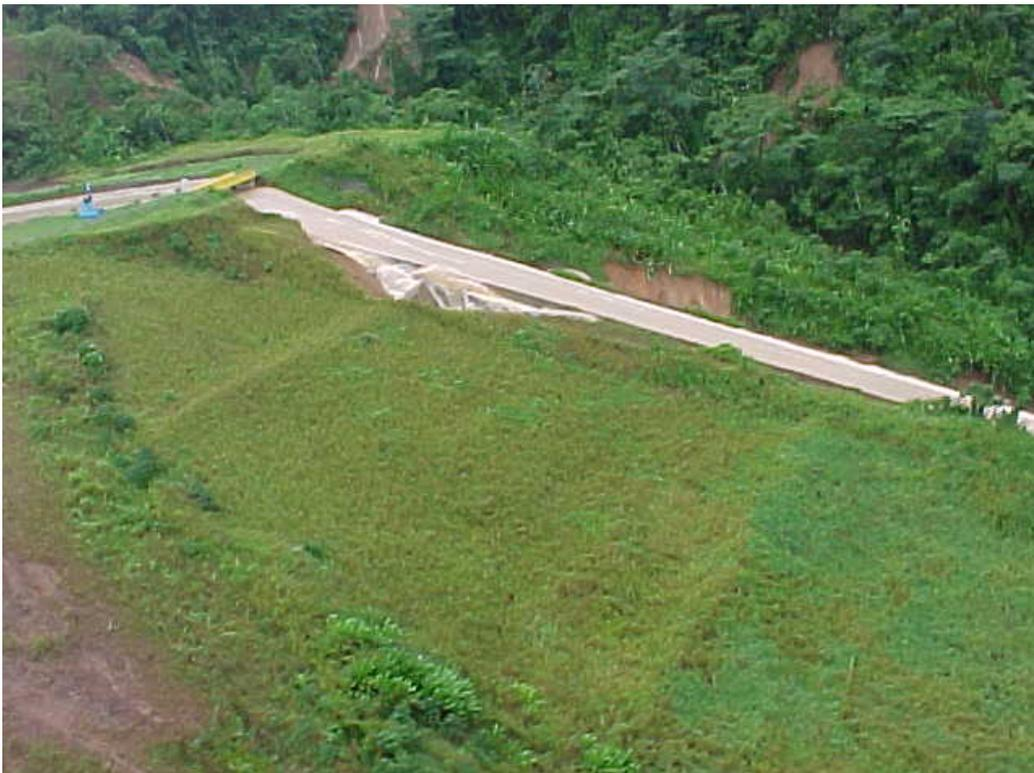
Figure 14: Overtopping Along Entire Length of Chute
