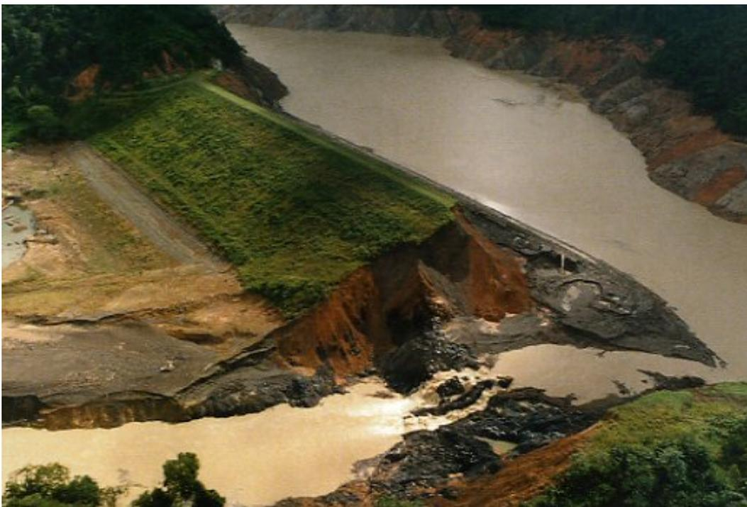
Figure 18: Aftermath of Reservoir Breach
