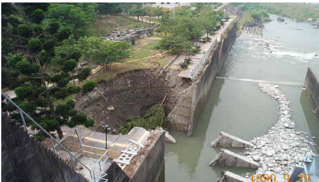
Figure 12: Failed Spillway Wall at Shih-Kang Dam
