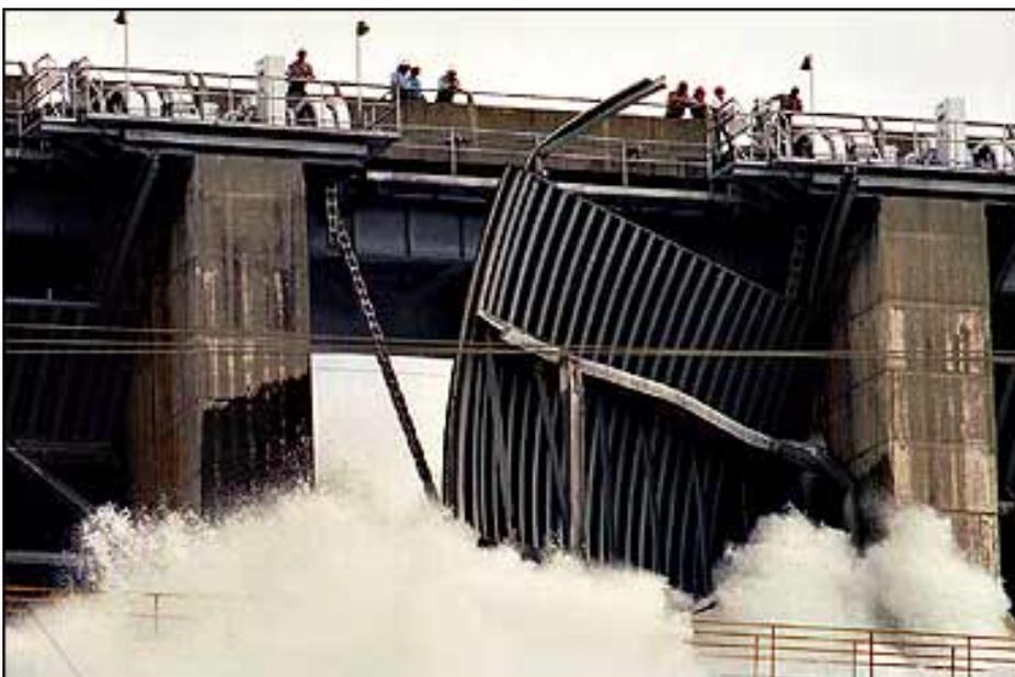
Figure 39: Folsom Dam radial gate failure
