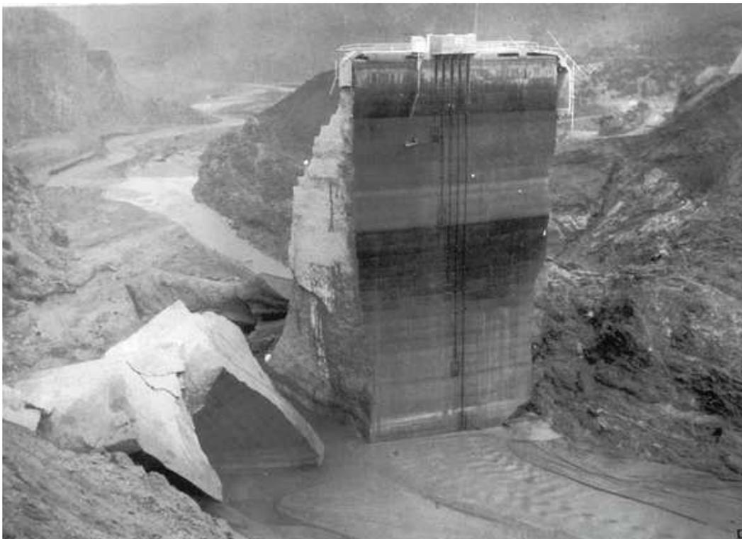
Figure 28: St Francis Dam after failure
