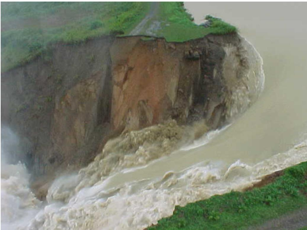
Figure 16: Headcutting Progressed to Reservoir
