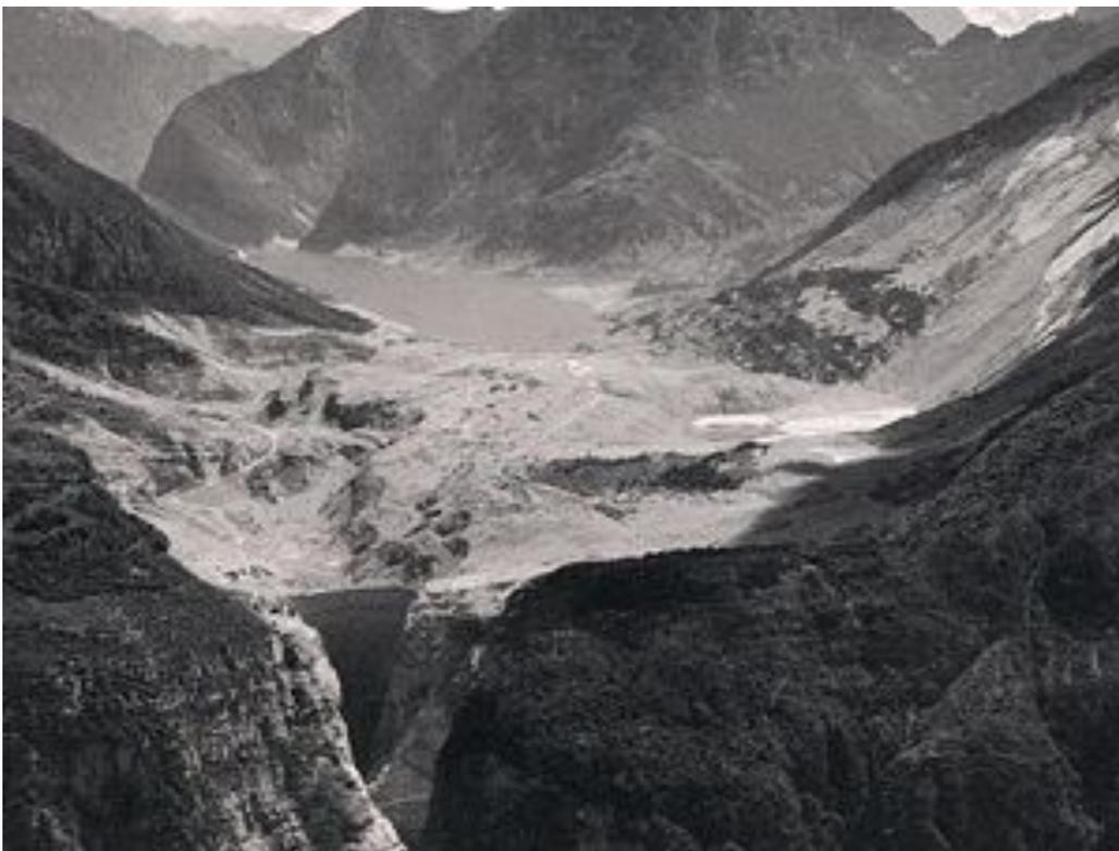
Figure 36: Vaiont Dam after the landslide
