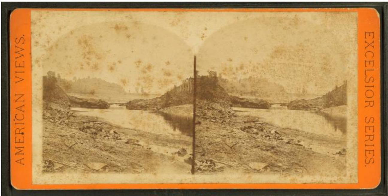
Figure 37: Stereoscope view of South Fork Dam after failure
