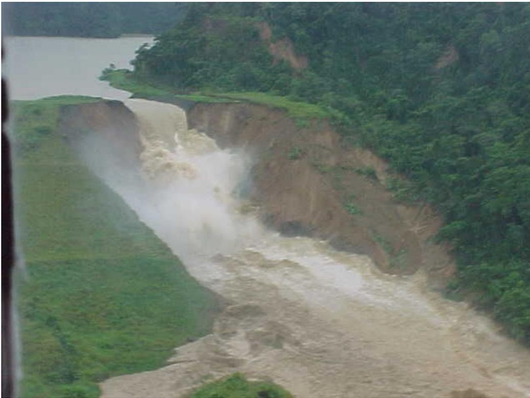
Figure 17: Breach Formation Nearing Completion
